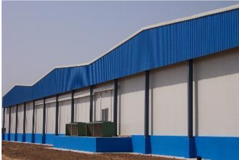
3. Anant Cold storage 150KW | Lucknow U.P.
