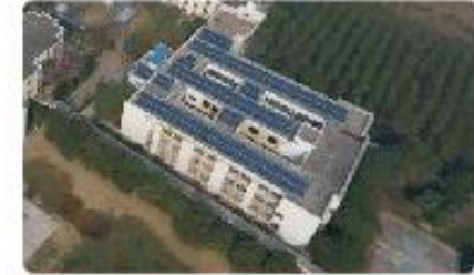
100kW PLANT AT JMIT, HARYANA
